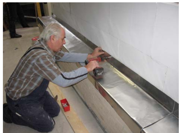
.....or fix direct into the wall with Hammerfix screw nails or SS fixings at 300mm centres.
