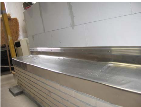
Fixation to the under surface. Use synthetic or SS steel strips.....
